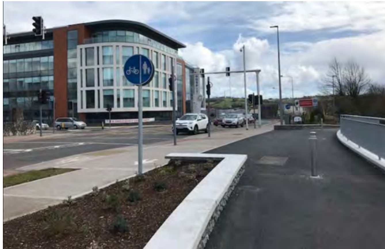
Figure 5.18: New Cycle Ramp access at junction of Mahon Link Road and St. Michael's Drive
