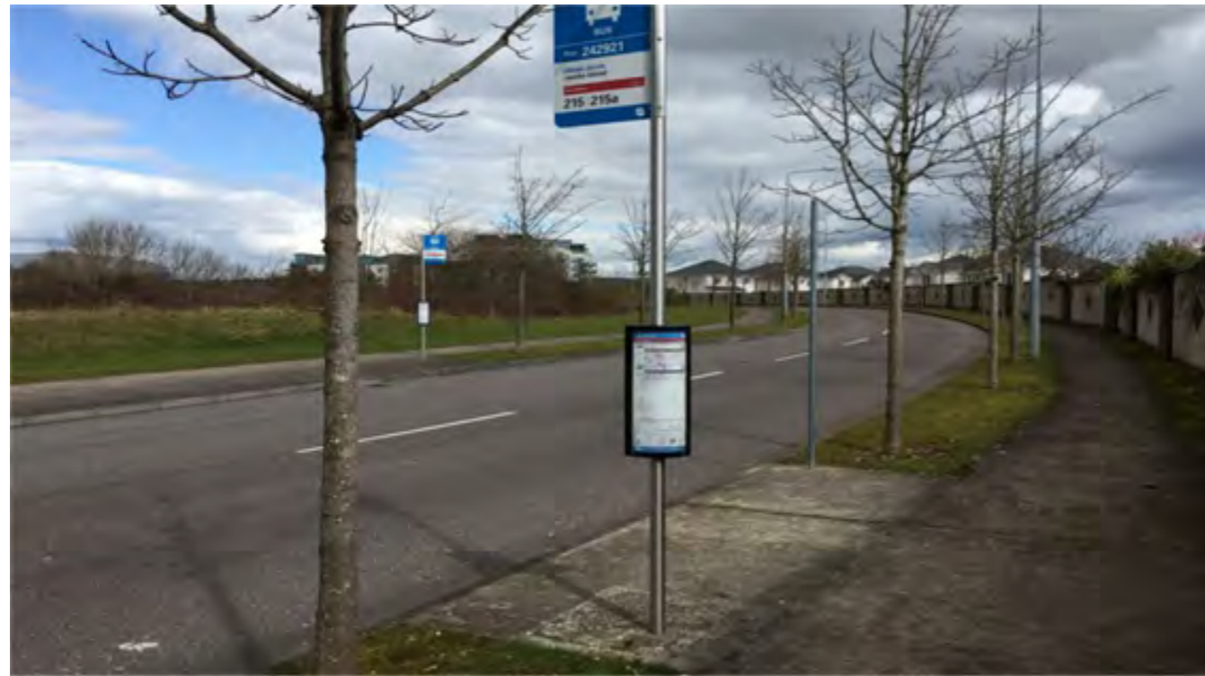
Figure 5.22: Existing Bus Stops on Jacob's Island internal spine road
