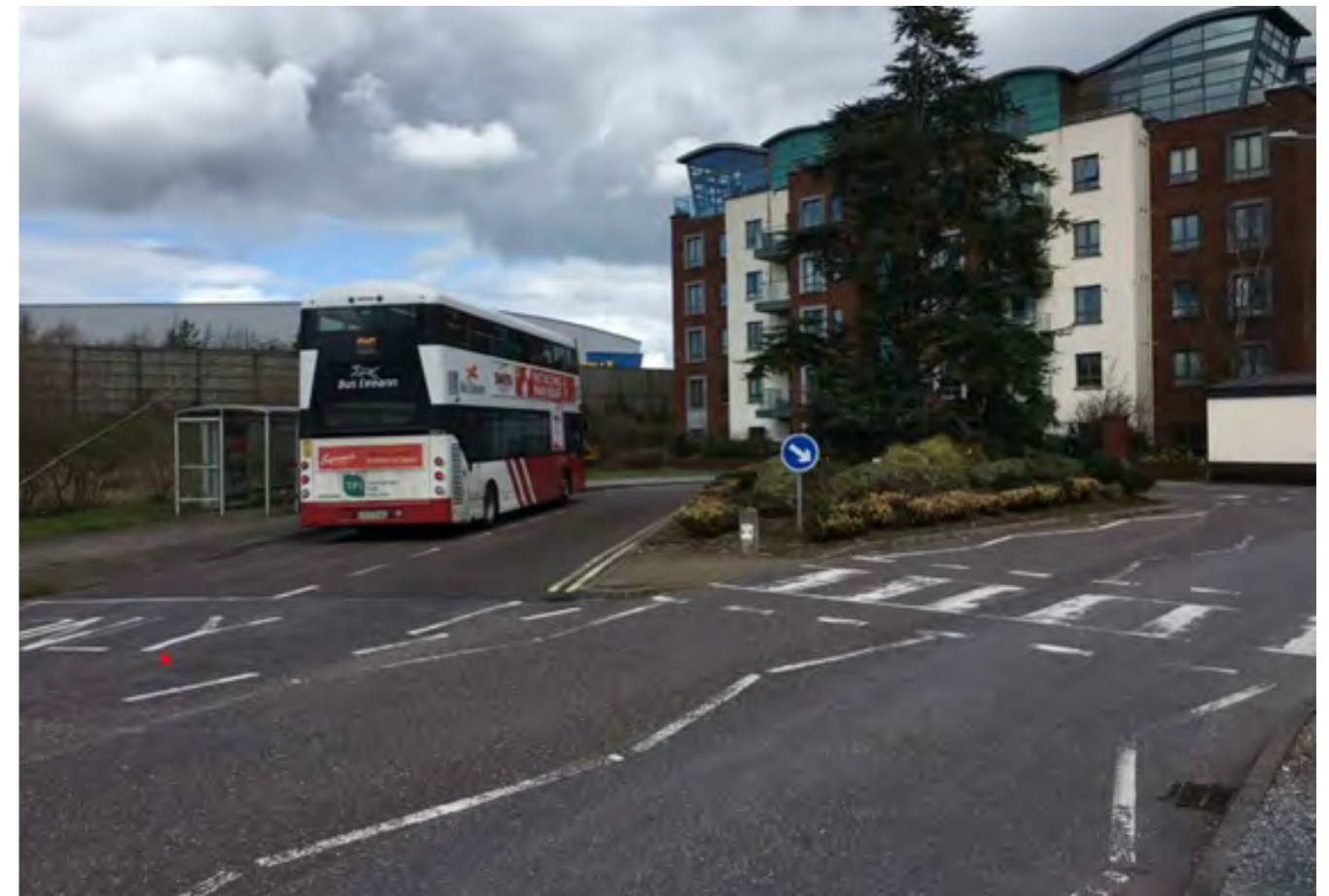
Figure 5.21: Existing Bus Terminus and Turnaround Area at The Sanctuary, Jacob's Island
