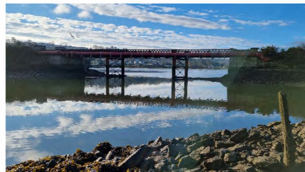
viii) Black Bridge facing south.
